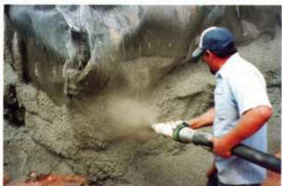
The C-30HDN is ideal for shotcrete applications of stiff, low slump mixes — swimming pools, ditch linings, soil stabilization, walls and more.
