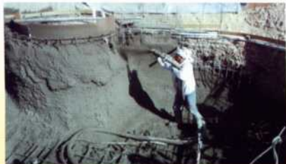
The ST-55, with its powerful ability to handle the toughest shotcrete mixes, enables a swimming pool contractor to apply shotcrete to two pools a day.
